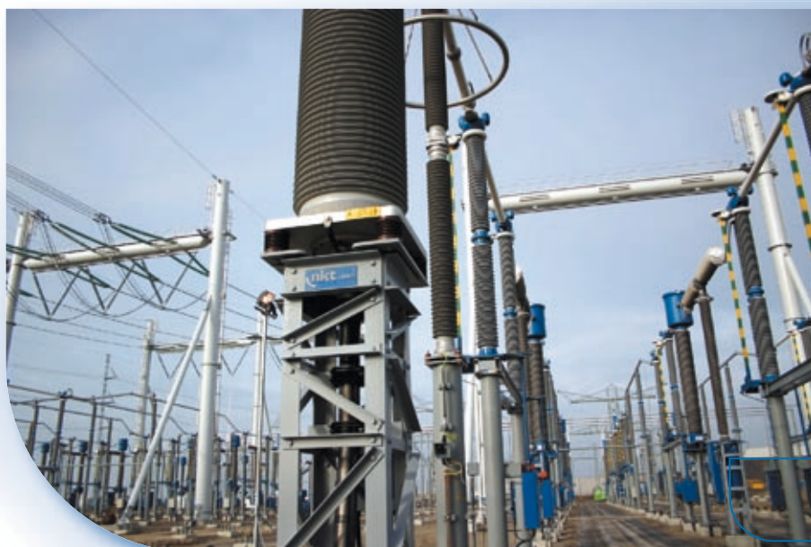
Outdoor Termination with Composite Insulator FEV 420-V
