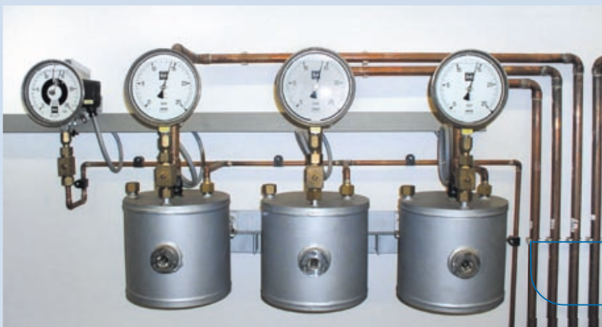
Oil Feeding Tanks for Low Pressure Oil Filled Cables
