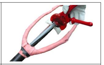
4.3 As each core is cut, apply temporary insulation to both core ends before starting on the next phase core. This temporary insulation consists of either a minimum of 6 layers of adhesive tape or an Approved tapered cap (secured in place with adhesive tape)
