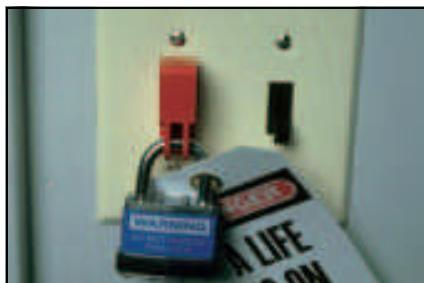
For locking out electrical supply controlled by ordinary toggle switches.
