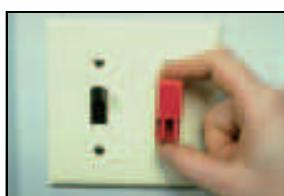
Turn switch to desired position. Place lockout over switch.
