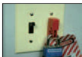
Attach padlock and tag. Test to insure secure lockout.
