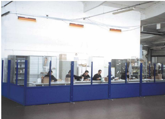
Fig. F – Partial heating with room dividers
