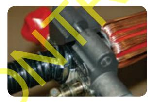
• Clean and degrease the insulation with an approved solvent wipe to remove all traces of conducting material. Always wipe from cut end towards screen wire to avoid contaminating the insulation with carbon from the uncut screen.
