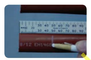
Using a sharp knife, cut around the core through the papers taking care not to damage the conductor below.
