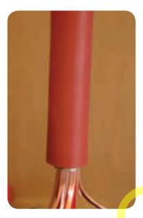
Use a soft yellow flame to shrink the red tube starting at the screen cut. Then shrink from the screen cut up to the cable lug, before finally shrinking from the screen cut to the bottom.
