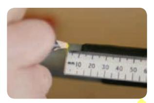
Make Chinagraph pencil marks on the black insulation screen of each core at 20mm, 40mm, 60mm and 90mm from the screen cut.
