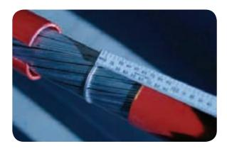
• Using a depth-guarded or junior hacksaw make a circular cut around the armours at the binder position. Cut through only half the width of the armour to avoid damaging the lead sheath below.
