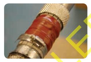
• Fit the metallic cage to the joint, overlapping the cage fingers fully onto the 'cheese-grater' area.
