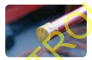
• Make a Chinagraph pencil mark on the insulation, 40mm from the cut end.
