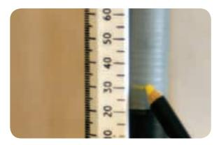
• Wrap the short piece of yellow mastic around the screen cut between the two marks. Stretch the tape to half its original width and form a smooth taper with no sharp edges.
