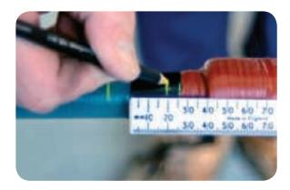
• Wrap the short piece of yellow mastic around the screen cut between the previously made marks. Stretch the tape to half its original width and form a smooth taper with no sharp edges.
