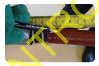
Make a second Chinagraph pencil mark 20mm onto the lead sheath.
