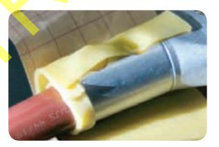
Wrap the yellow mastic patch around the single end of the connector, leaving the outer backing sheet in place to prevent other patches sticking to it.
