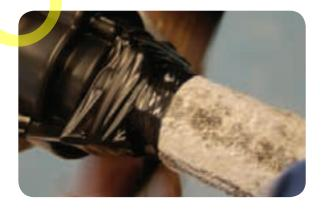
For extra security, run a length of PVC tape down the seams of the joint shell and fit the plastic lid.
