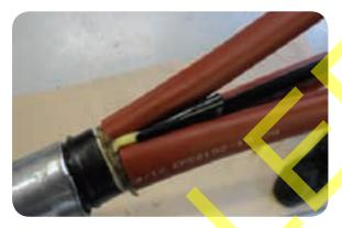
Remove the PVC Tape from the belt papers and make a Chinagraph pencil mark on the red tubes 40mm from the lead sheath cut.
