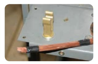
• Cut each bunch of copper wires to the correct length using the installed mechanical connector as a guide.
