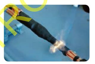
Apply additional heat over the connector to ensure that the tube is fully shrunk and wrinkle free. The second picture below shows what the finished tube should look like.
