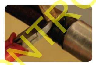
Carefully separate the cores and secure the core paper ends with PVC tape.
