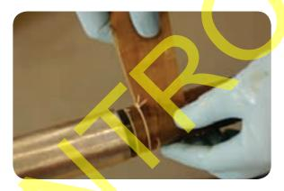
• Install five layers of PVC tape over the prepared belt and carbon papers, sticky side out, to avoid damaging the papers when the fillers are removed and the heatshrink tubes are fitted.
