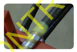
• Slide the correct lengths of red insulating tube over each core, until they are approximately 50mm from the crutch.
