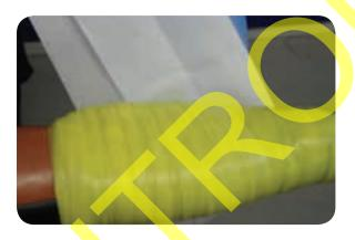
Lubricate the yellow mastic with the supplied silicone tissue to stop the black stress control
