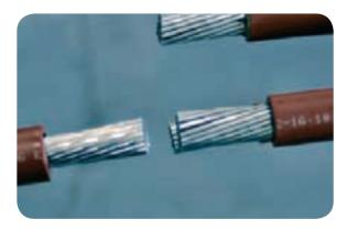
Insert each end of the core into its respective 'connector half' and finger-tighten the bolts.
