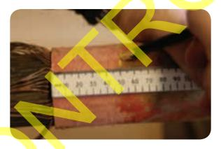
• Wrap a one-third-lap layer of red sealant tape around the sheath up to the Chinagraph pencil mark.
