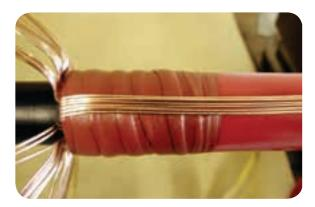
• Apply a double wire binder to the screen wires level with the end of the red sealant tape.
