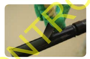
Repeat this operation for the remaining section of insulation screen.
