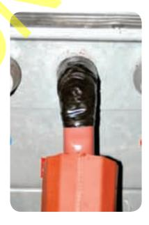
• Push the boots up and over the bushings as far as they will go. Begin shrinking each boot in place with a soft flame, starting at the inside leg/body interface, before moving up the bushing. Finally shrink from the centre of the boot down to the bottom of each leg.
