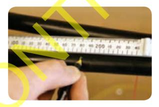
• Apply six turns of PVC tape, sticky side out, to the insulation screen to provide a guide for the abrafile.
