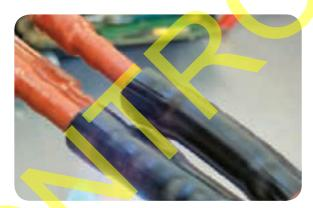
• Remove the heat from that end and start shrinking from the middle again towards the other end, stopping again 50mm from the end. This ensures that as the tubes shrink any air inside is pushed out.
