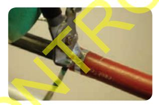
• Fix the tinned copper braid fixed to the 'cheese-grater' to the outer sheath of the cable 60mm from the sheath cut.
