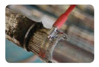
• Fold a length of copper mesh in half over its full length so that its width is reduced to 30mm. Wrap the mesh around the lead sheath level with the end of the red crutch tube.
