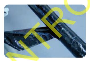
Apply more heat to the final layer of bitumen on the lead sheath and armours and wipe off any traces of bitumen with approved solvent wipes.
