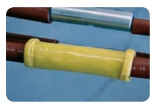
• Slide the red and black insulation tube over the installed yellow patch and position over the centre of the joint. Position all three before starting the shrinking process.
