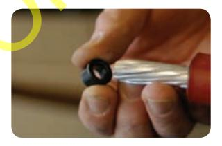
• Place the black stress-control tube inside the red and black insulation tube and park it on the single cable end. Insert the single cable into the connector and finger-tighten the bolts.
