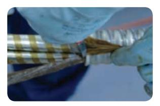
Rewind the CWT tightly around the cable cores at the crutch position for a distance of 20mm from the aluminium sheath cut and tie off and remove any surplus tape with insulated side cutters.
