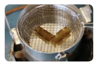
If the wax froths a lot and makes a crackling noise, this means that the papers are wet and the cable is not to be jointed.
