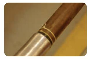
Carefully unwind two or three of the belt papers at a time and tear them off neatly against the twine binder.
