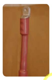
• **Note:** After installing the termination, reheat the cable lug area until a bead of green mastic appears at the top.
