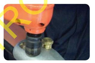
• If any of the bolts shear off proud of the connector surface, remove the edge with a file.
