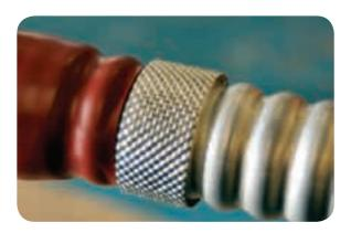
• Fit the metallic cage to the joint, overlapping the cage fingers onto the 'cheese-grater' area.
