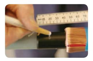
Make a second Chinagraph pencil mark on the insulation 10mm from the screen cut.
