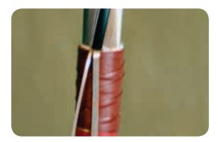
Apply a double wire binder to the screen wires level with the end of the red sealant tape.
