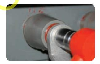
Now push the boot upwards and over onto the bushing as far as it will go. When installed it shall not be more than 15mm away from the back plate of the end box.
