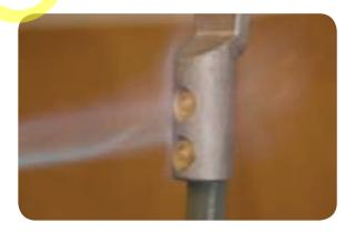
• Place the green-mastic-lined red tube on the termination until the bottom is level with the wire binder.
