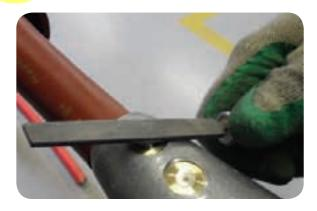
Clean and degrease the connector, fill the bolt holes with the supplied clay pack to obtain a smooth finish.
