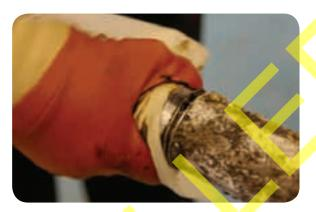
Place a wire binder around the tape armour 60mm from the outer serving removal point.
