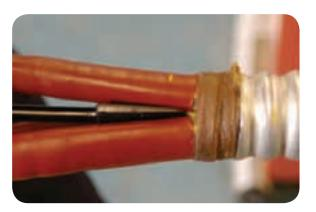
• Make a Chinagraph pencil mark on the red tubes 40mm from the aluminium sheath cut.
