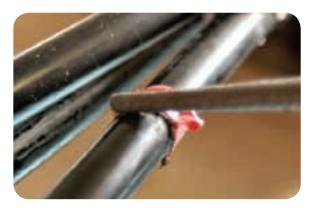
• Remove the PVC tape. Use a 0.4mm depth-guarded tool to make two separate score lines along the core from the screen cut to the cut end. The lines shall be equally spaced and approximately 30° apart.
