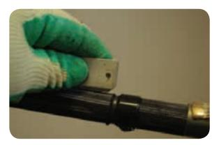
• Where the score meets the cut end, further deepen the score marks and pull the conducting screen away from the insulation up to the circular abrasion.
