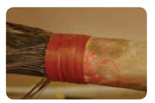
• Fold the copper wires back onto the red sealant tape and secure them with a double wire binder, level with the end of the mastic.
