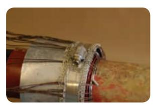
• Trim the copper wires with side cutters, so that they are level with the inner end of the copper wire mesh.
