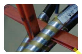
Wrap a 50mm long piece of yellow mastic, stretched to half its original width, around the screen cuts between the two Chinagraph pencil marks.
