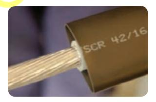
Shrink the tubing down starting at the insulation cut, then work back towards the cable over sheath.
