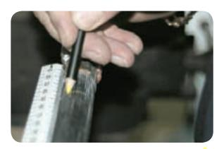
Apply six turns of PVC tape to the insulation screen, sticky side out, to provide a guide for the abrafile.
