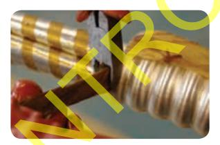
• Rewind the CWT tightly around the cable cores at the crutch position for a distance of 20mm from the aluminium sheath cut and tie off. Remove any surplus tape with insulated side cutters.
