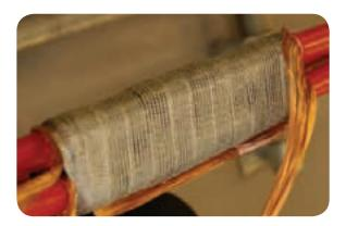
Cut one bunch of copper wire screens in the centre of the joint and fit into one half of the
