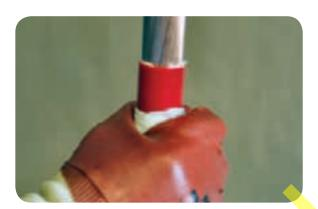
Make a Chinagraph pencil mark on the outer sheath of the cable, 60mm from the sheath cut.
