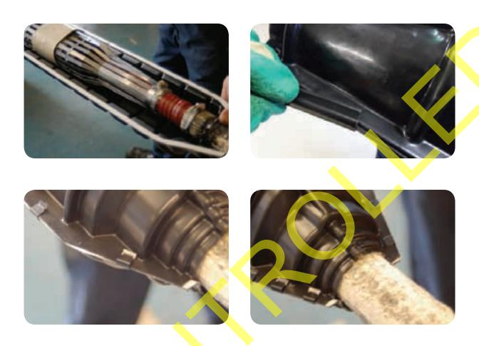
Tape the joint box to the incoming cable with PVC or another suitable tape. If necessary, pack the ends of the joint shell out with the clay pack supplied in some kits.
