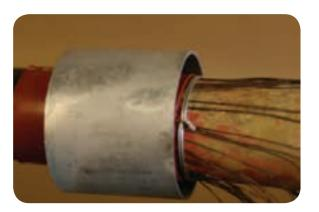
• Fold a length of copper mesh in half over its full length to reduce its width to approximately 30mm. Wrap two layers of the mesh around the edge of the support ring (furthest away from the joint) and temporarily secure.
