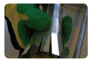
Dress down the earth strip fingers onto the copper mesh, over the lead sheath and armours area at the other end. Secure the earth strip in this position with a double binder around the centre.
