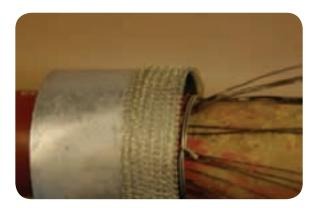
• Turn back the copper wires and lay them over the copper mesh so they are tidy and do not cross each other.
