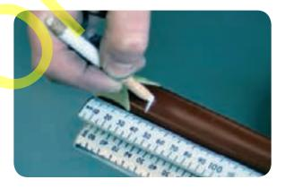
Apply another short piece of yellow mastic, stretched to half its original width, between the Chinagraph pencil mark and the end of the core
