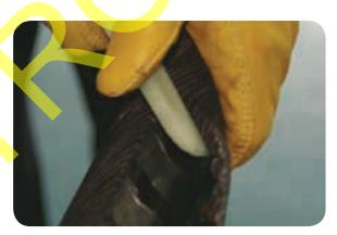
Unwrap the bedding and remove it using an approved knife. Take care not to damage the cores below.
