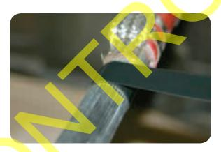
• Using an abrafile, make a circular abrasion around the screen at the removal point just deep enough to expose the insulation below.
