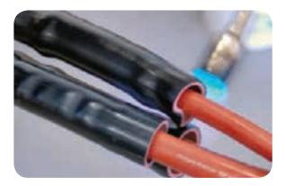
Return to each end in turn and continue to shrink the tubes completely.
