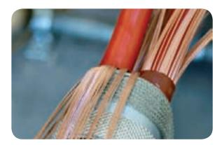
Wrap the remaining copper mesh over the wires and secure with a half hitch. Clamp the
