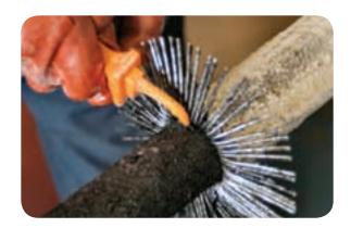
• At the open cable end lift the bitumen impregnated textile layer with the knife and unwrap it back to the armour position, tearing it against the end of the cut armours. The use of a gas torch assists this process.
