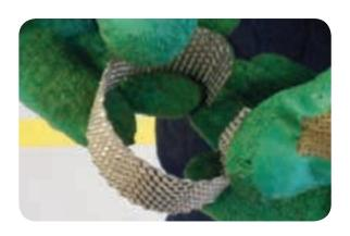
• Install the 'cheese-grater' strip next to the red crutch sealing sleeve, ensuring that it bridges two adjacent peaks on the corrugated aluminium sheath.
