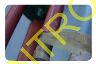
Clean any surplus compound from the cable conductor with an approved solvent wipe.
