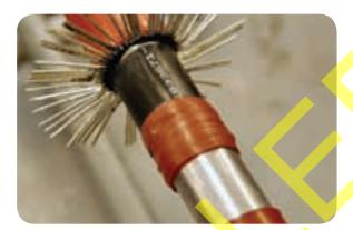
• Fold a length of copper mesh in half over its full length, so that its width is reduced by half, and wrap it around the lead at the end of the black sealing sleeve.
