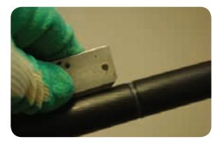
• At the position where the scores meet the cut end, further deepen the score marks and pull the conducting screen away from the insulation up to the circular abrasion. Repeat this operation for the other screen section.
