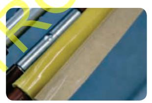
• Roll the overlapped ends of the yellow mastic patch over to help with filling the gap between the edge of the connector and the core tubes. Complete this stage for all three cores before attempting to shrink the red and black insulation tubes in place.
