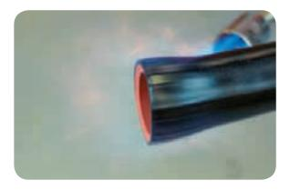
Return to each end in turn and continue to shrink the tube completely.
