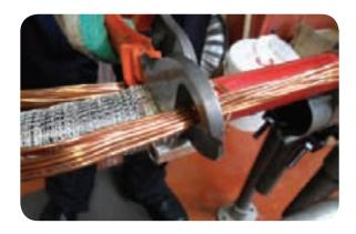
Insert each bunch into each of the connectors and shear off the second bolt.
