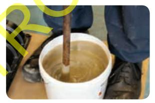
Pour the mixed resin into the joint shell.
