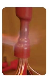
The termination is now ready to be installed in the end box.
