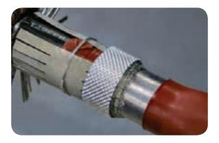
• Fold another length of copper mesh in half over its full length, so that the width is reduced by half, and wrap it around the fingers on the armour end of the clip.
