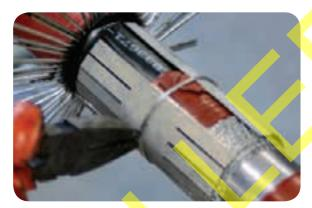
Fold a length of copper mesh in half over its full length, so that the width is reduced by half, and wrap it around the fingers on the lead sheath end of the clip.
