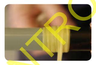
• Slide the black stress control tube over the core until the end is level with the insulation cut. The tube shall fully overlap the yellow mastic tape.
