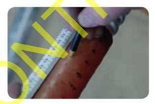
• Abrade the PVC sheath with a rasp between the sheath cut and the Chinagraph pencil mark.
