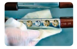
• Remove one of the backing sheets from the yellow mastic patch and position it underneath the connector, so it is in the centre of the sticky side and the overlap is over the bolt holes.
