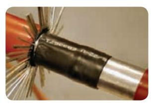
• Apply two layers of red sealant tape over the black sealing sleeve for 40mm, starting at the end nearest to the lead sheath and working towards the armours.
