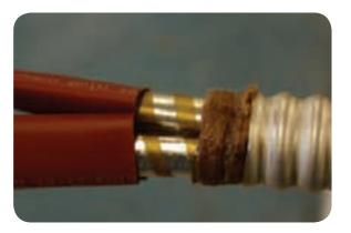
Partly shrink the tubes for a distance of 50mm from the end. Whilst the tubes are still hot, gently twist and turn them so that the shrunk section is positioned on the inside and the ends of the tubes are level with the CWT tape protecting the belt papers.
