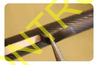
Clean and degrease the insulation with a solvent wipe to remove all traces of conducting material. Always wipe from the cut end towards the screen wire to avoid contaminating the insulation with carbon from the uncut screen.
