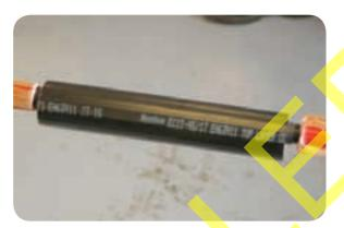
• Starting in the middle, shrink the insulation tube using equal heat on all the surfaces. When the tube is properly shrunk, the ridges on the black layer of the tube shall no longer be visible and the tube cannot be moved.
