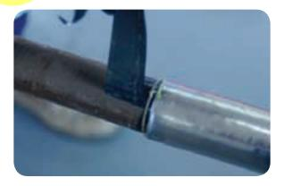
• Now tie a second twine binder around the belt papers 20mm from the aluminium sheath cut.
