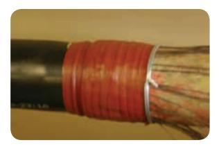
Push the large red crutch sealing sleeve from the transition joint kit over the cable end and line it up with the wire binder. Shrink into place starting from the wire binder end.
