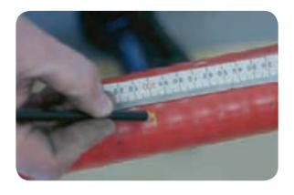
Cut round the sheath at both of these marks using a pair of PG4 sheath stripping pliers.
