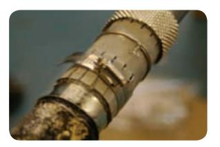
• Apply two one-third-lap layers of red sealant tape on the earth strip between the 'cheese-grater' and the worm drive clip at the armour end.
