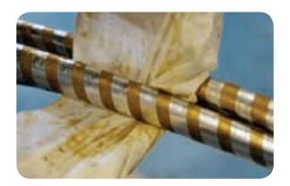
Mark the screen papers at the removal point indicated on the relevant jointing instruction.
