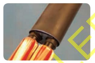
Shrink the stress control tube down, starting at the branch side before working towards the single core side.
