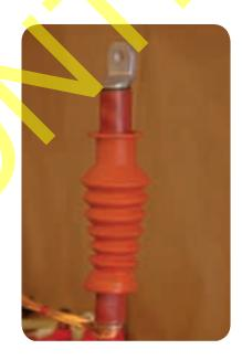
• Apply a thin layer of silicone grease to the top 50mm of the termination.
