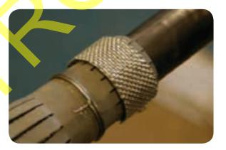
Fasten the other ends of the fingers onto the armours using a worm drive clip.
