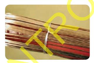
Make a Chinagraph pencil mark on the insulation screen 15mm in from the sheath cut.
