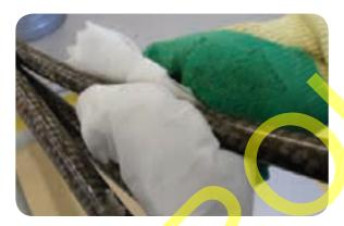
Tape up the paper insulation on the end of each core to stop them unravelling.
