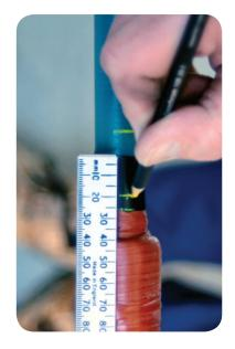
Make a second Chinagraph pencil mark on the insulation 10mm from the screen cut.
