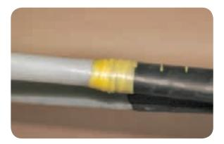
Apply one turn of red sealant tape around the semi-conducting screen of each core between the third and fourth Chinagraph pencil marks.
