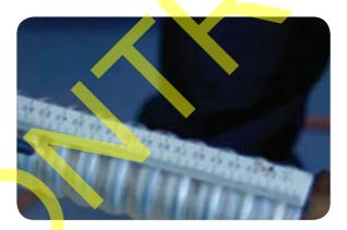
• Using the approved tool, make a circular cut around the marked ridge of the aluminium sheath. The cut should be right through the aluminium. Take care not to damage the papers below.
