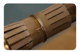
• Fold the remaining copper mesh roll in half lengthways. Wrap it around the end of the earth strip over the lead sheath end. Form the 'cheese-grater' strip into a circle and fit it over the mesh.
