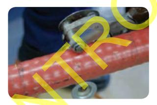
• Lift the edge of the sheath with the jaws of the PG4 Pliers and unwrap it, tearing against the circular cut points. Gentle heat from a gas torch may assist this operation in cold weather.
