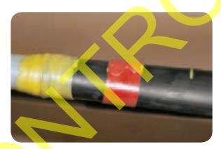
• Carefully slide the red core tubes over the end of each core until the tubes are level with the fifth Chinagraph pencil mark.
