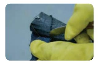
Apply sufficient heat to the inner bitumen paper layer to soften it before removing it.
