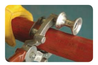
From the open end of the cable make a longitudinal cut down the sheath to the circular cut mark. Remove the sheath at this mark by unwrapping from the armours or screen wires below.
