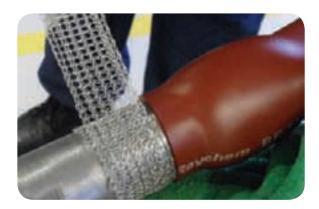
• Trim the 'cheese-grater' strip to length and form it into a circular shape, so that it fits neatly and securely around the copper mesh.
