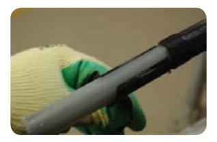
Carefully remove the PVC tape. Clean and degrease the insulation with an approved solvent wipe to remove all traces of conducting material. Always wipe from the cut end towards the screen wires to avoid contaminating the insulation with carbon from the uncut screen.
