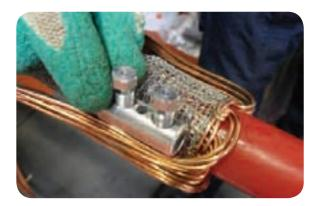
• Shear off one bolt on each connector, ensuring that space is left in the connector to fit the rest of the copper wires in the other end.
