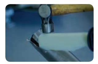
Open the lead sheath up along the length of the cut and carefully unwrap the lead sheath against the round cut.
