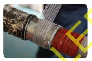
Lay a red sealant tape strip down the centre of the tinned copper strip with fingers at each end. This is an important moisture seal and shall not be left out.
