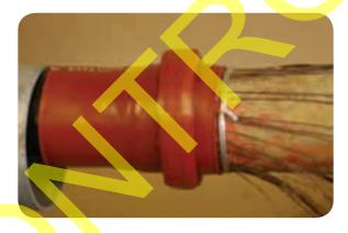
Place the support ring over the mastic and line the end of it up with the double wire binder.
