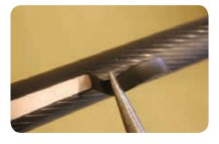
Clean and degrease the insulation with an approved solvent wipe to remove all traces of conducting material. Always wipe from cut end towards screen wires to avoid contaminating the insulation with carbon from the uncut screen.
