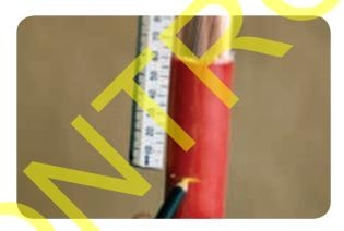
• Wrap a one-third-lap layer of red sealant tape over the cable sheath down to the Chinagraph pencil mark.
