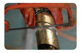
• Lift the point of the armours at the binder position, unwrap and remove.
