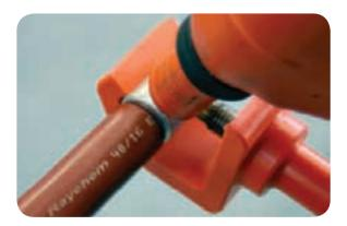
Repeat this operation on the other side of the connector, then shear off the central fixing bolt.
