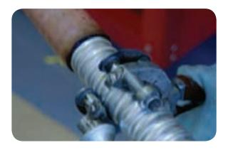
Once the circular cut has been made, the aluminium sheath can be removed by pulling the sheath towards the open cable end. Twisting the sheath from side to side whilst pulling shall make this task easier.
