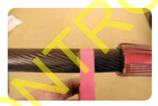
• Use an abrafile to make a circular abrasion around the screen, using the PVC tape as a guide, just deep enough so that the insulation below is visible.
