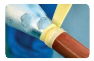
• Fill in the gaps between the core and the connector, continuing across the connector and on to the red insulating piece. Ensure that a smooth profile is formed so that when the heat shrink tubes are applied all the voids are filled with yellow mastic.
