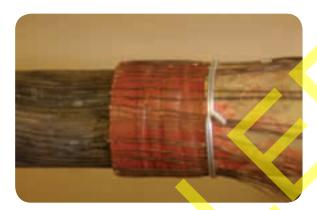
Place the piece of black heatshrink tube supplied in the 3 core polymeric preparation kit over the inner bedding layer of the cable and shrink into place.
