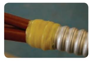
• Position the red crutch sealing sleeve centrally over the yellow mastic, sheath and red tubes, and then shrink into position. Apply sufficient heat to ensure that the tube has been fully shrunk, thus making sure that the yellow mastic fills any voids in the crutch area.
