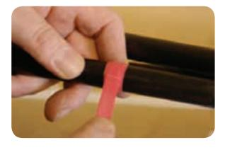
• Use an abrafile to make a circular abrasion around the screen at the removal point, just deep enough to expose the insulation below. Take extra care on cables with sector-shaped cores to ensure that only the minimum amount of insulation is removed.
