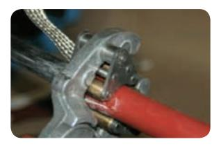
• Install the first ligerex strap around the cable sheath, 5mm back from the sheath cut, and secure with the ligerex tightening tool.
