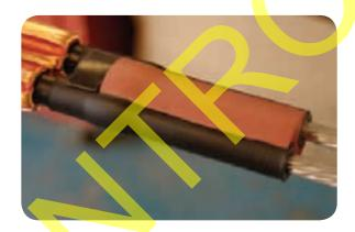
• Fit the two conductors into the mechanical connector, ensuring that the insulation edge butts against the connector body. Tape the two cables together with the supplied tape to stop the inserts falling out.
