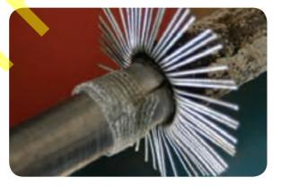
Bend the steel wire armours back down and secure in place with the worm drive clip supplied in the kit.
