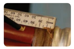
Make a second Chinagraph pencil mark 20mm onto the aluminium sheath.
