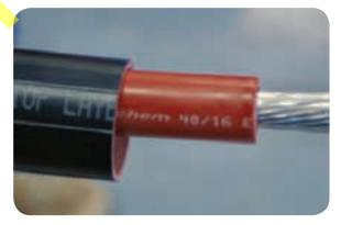
• Set the cores in their final jointing position. Ensure that the conductors have been cut to allow for the connector central moisture block.
