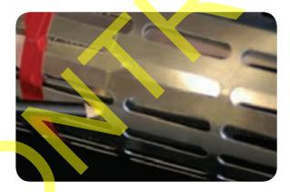
• Remove the backing from the rubber patches supplied in the kit and apply centrally, sticky side out, over the Chinagraph pencil marks on the aluminium cage. Ensure that any mechanical earth connectors are pulled tight into the mesh.
