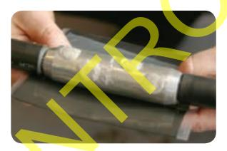
Wrap the black mastic patch around the connector and remove the other backing sheet.
