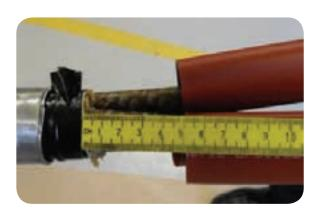
• Partly shrink the tubes for a distance of 50mm from the end.
