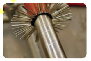
Apply two half-lap layers of red sealant tape for 40mm between the two Chinagraph pencil marks.
