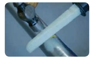
• From the cut cable end, cut the lead sheath longitudinally to the round cut, using an approved insulated hack-knife. Take care not to damage the belt papers below.
