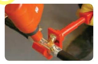
• Continue to tighten and shear off all four bolts, starting with the bolts at either end of the connector, followed by the two in the centre.
