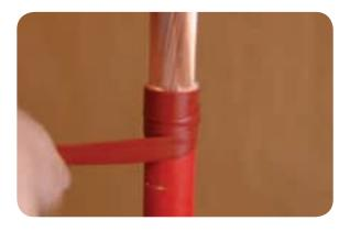
Bend back the screen wires and lay them onto the mastic tape taking care not to cross over any of the wires.
