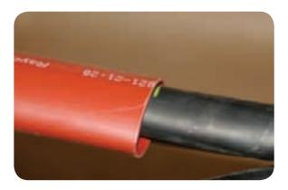
Shrink the tubes down starting at the insulation screen cut end before working towards the cut cable end.
