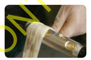
• Fill the bolt holes in the mechanical connector with the grey clay material supplied in the joint kit.
