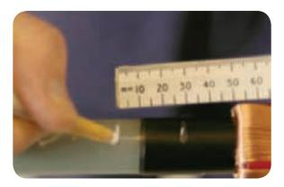
• Stretch one of the short yellow mastic strips, supplied in the kit, to half its original width and wrap it around the core screen and insulation between the two Chinagraph pencil marks.
