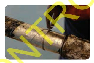
Wear suitable gloves while removing the armour. Using a depth-guarded or junior hacksaw, cut through the first layer of tape armour at the binder position.
