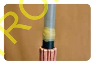
Preheat the cable lug before placing the red tubing over the core.
