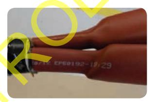
Continue to shrink the tubes starting from the crutch and working towards the cut ends.
