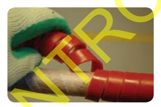
• Remove the fabric or plastic tape from the screen wire using an approved knife, taking care not to damage the copper wires below.
