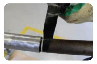
Now tie a second twine binder around the belt papers 20mm from the lead sheath cut.
