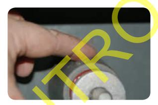
Bolt the lugs to the bushings using the nuts and bolts supplied with the switchgear. Tighten
