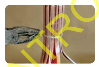
Make a Chinagraph pencil mark on the black insulation screen of the cable, 20mm from the screen cut.
