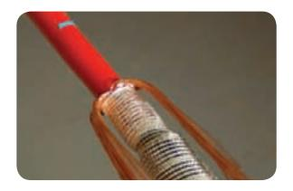
Using one of the tinned aluminium connectors as a guide, cut the copper wire screens to length so that the connectors sit in the gap between the wire binder and the end of the insulation tube.
