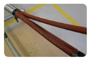
• Whilst the red tubes are still hot slide the supplied yellow mastic wedge into the crutch so that the tip is just below the belt paper. The yellow mastic wedge shall be applied with a thin coating of silicone grease and a plastic wedge insertion tool.
