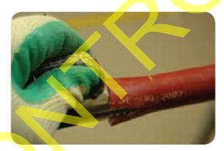
• Use the sheath roller tool to compress the sheath on to the serrations of the 'cheese-grater', until the sheath is back to its original position.
