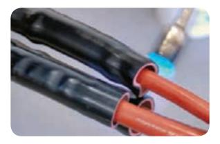
Return to each end in turn and continue to shrink the tubes completely.
