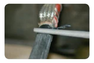
• Starting at this position, and using the correct 0.6mm depth guarded tool, make two separate score lines along the core towards the cut end. The lines shall be equally spaced and approximately 90° apart.
