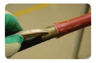
• Ease the sheath outwards, carefully progressing around the sheath in a circular pattern until it is approximately between 5mm and 7mm above its original position. Do it gently to avoid cracking the aluminium layer which reduces its fault carrying capability.
