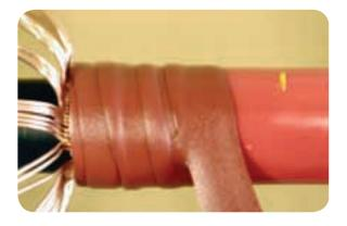
Bend back the screen wires and lay them onto the mastic tape, taking care not to cross over any of the wires.
