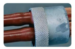
• Fold a length of copper mesh in half over its full length so that its width is reduced to approximately 30mm. Wrap two layers of the mesh around the edge of the support ring (furthest away from the joint) and temporarily secure them.
