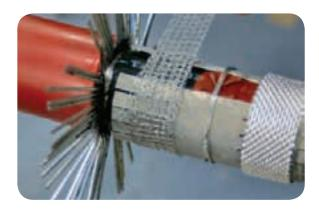
• Now lay the armours down over the copper mesh and secure them with the worm drive clip supplied in the kit.
