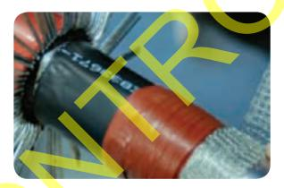
Remove the backing paper from one piece of red sealant tape and stick it down the centre
