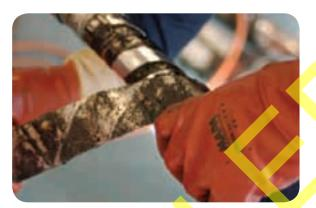
Repeat the process with the second layer of tape armour making sure not to damage the lead sheath below.
