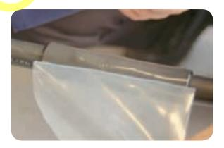
Slide the red and black insulation tube over the installed black patch and position it over the centre of the joint.
