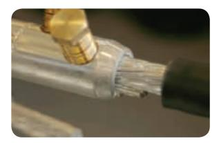
• Fit the conductors into the connector. The insulation butts up against the end of the connector.
