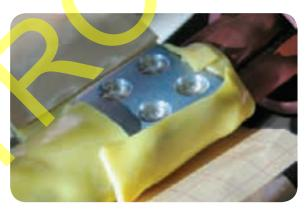
• Remove the backing sheet partly from the yellow mastic patch on the top of the connector and continue to wrap it around the connector until it is evenly covered.
