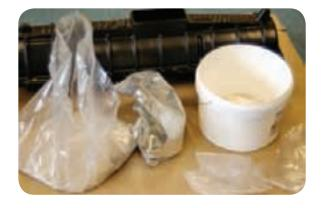
• Pick up the foil bag containing the resin and hardener. Apply pressure to the large resin pouch so that the resin breaks the seal between the two sections and mixes with the hardener.
