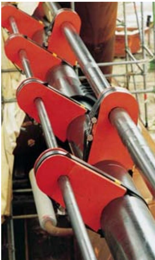
Epoxy Composite Clamps and Kevlar Straps
