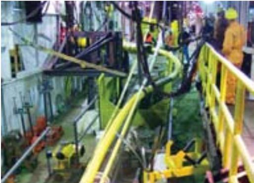
Piggyback Blocks being installed on Lay Barge
