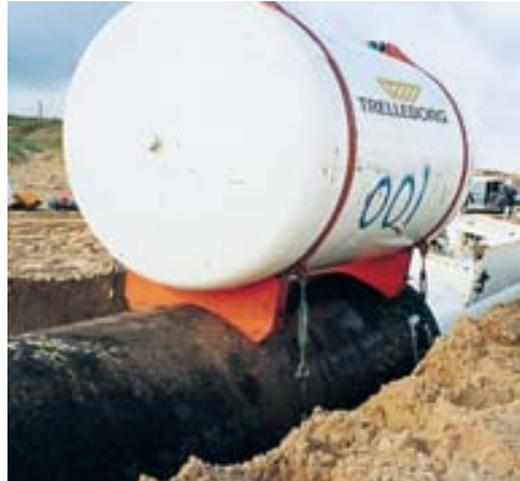
Pipeline Interface Saddles for Buoyancy Tanks
