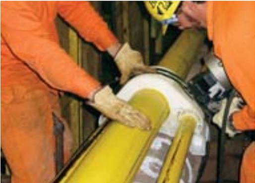
Banding being installed onto the blocks on the Lay Barge
