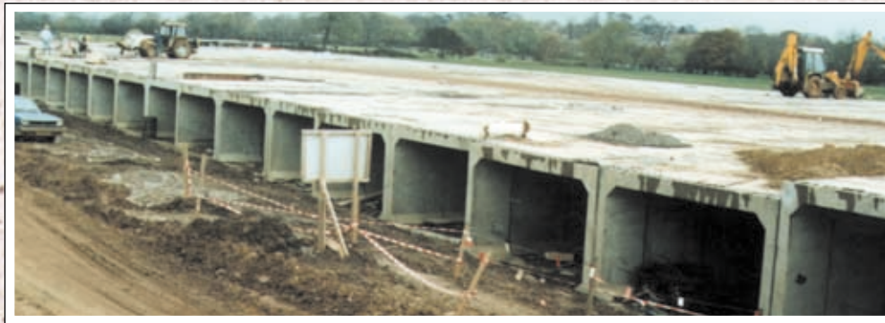
A large water storage project incorporating box culverts jointed with Tokstrip.
