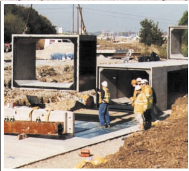
A box culvert unit is lowered into position.
