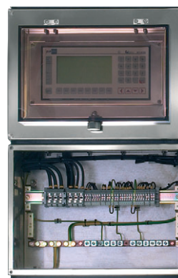
Terminals of different sizes on standard terminal rails, fitted PE- and N-rails
