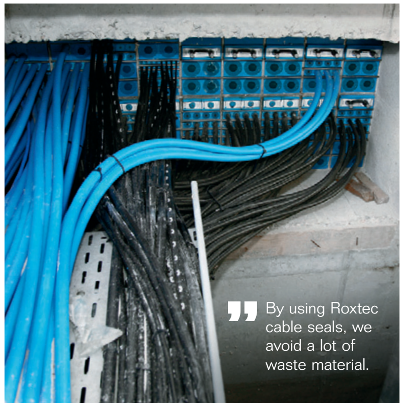
Gas-tight Roxtec seals between basements and concrete cable ducts.
