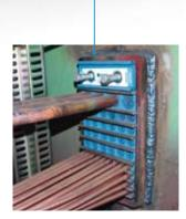
Roxtec S 6x1 for pressure-proof passage of copper pneumatic pipes in bulkheads onboard an FPSO.
