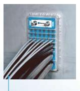
Roxtec RS entry seals securing weather tight installation of cabling to external lamps of a drilling rig.
