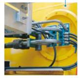
Roxtec S 6x2 for weather proofing and vibration dampening in machine room wall of offshore crane on a production platform.
