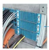
Roxtec G 8+8x3 transit for fireproof installation in refinery between outside to inside of control room.
