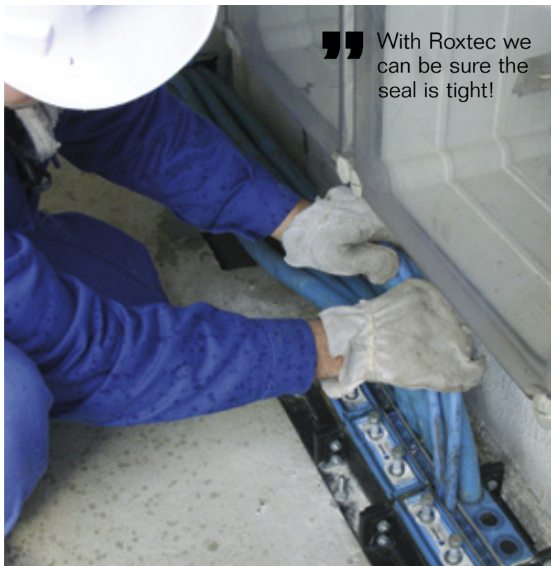
Roxtec seals cables in a manhole outside of the control room. Spare capacity has been added with extra seals for future cables.
