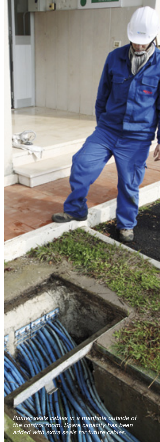
Cable transits into the auxiliary service room sealed with Roxtec.
