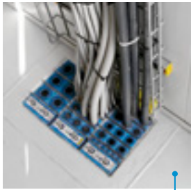
Transits between fire zones in offshore substations.
