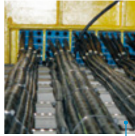
Deck transits for instrumentation.
