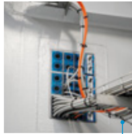
Transits between fire zones in offshore substations.
