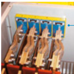
Bus bar transits for transformer room.
