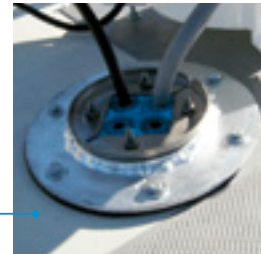
Transits for hub, radar, weather station and aeronautical obstruction lighting.
