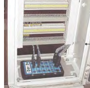
KFO frame in signalling cabinet
