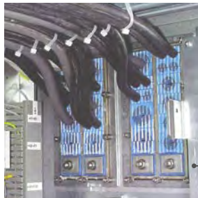
CF 32 with shielding protection in signalling cabinet
