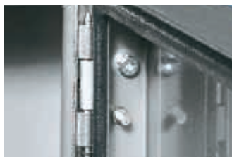
PE conductor connection point in the door.
