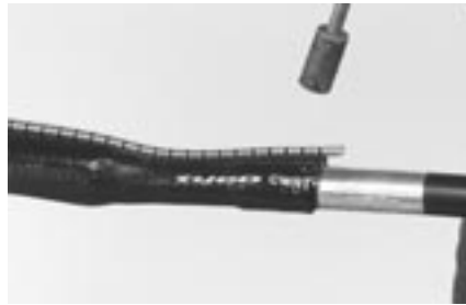
20 Postheat the rail and channel area at the sleeve end for approx. 30 seconds.
