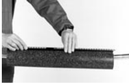
17 Pull the flexible channel over the sleeve rails until they butt on top of the underclip. Centre the sleeve over the splice such that the ends match the blue line of the cable aluminium foil.
