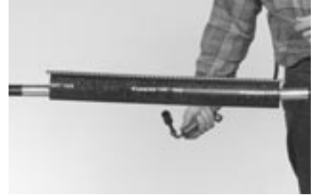
18 Start heating in the center of the sleeve, opposite from the channel. Then shrink the closure circumferentially through the center and continue to one end. Turn all the temperature indicating paint to black as you go.
