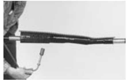
21 Continue heating the sleeve, starting again from the centre to the other end. Repeat steps 19 and 20.
