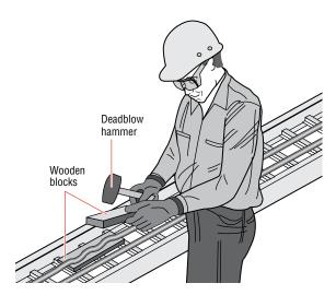
Figure 8: Straightening and dressing MI cable
