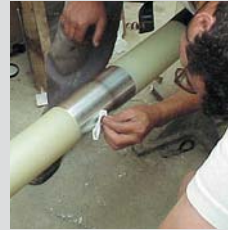
Cable core finishing
