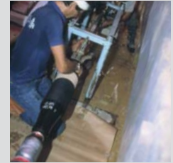
Joint sleeve positioning
