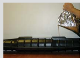
Pouring of polyurethane resin
