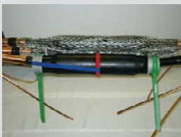
Joint body in position
