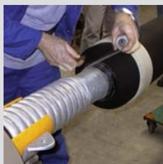
JOINT CORE FINISHING
