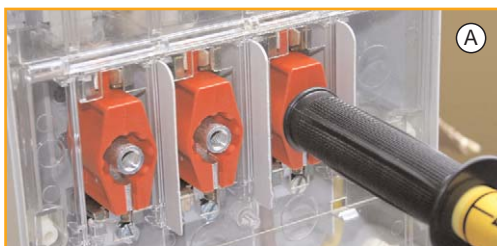
Installation of phase connection parts
