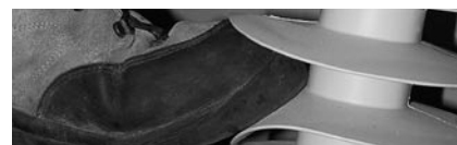
Fig. 34: Climbing on insulators is prohibited
