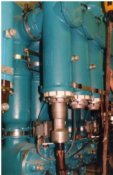
Figure 5: GIS Siemens Type 8DN9 with High-Voltage cable termination system and IEC extension adapter.
