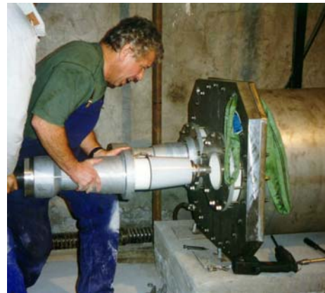
Figure 15: Plugging in the cable termination system to a T-Joint at BPSB Xian (China).
