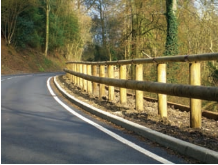
Timber faced safety barrier in forest area with optional handrail.
