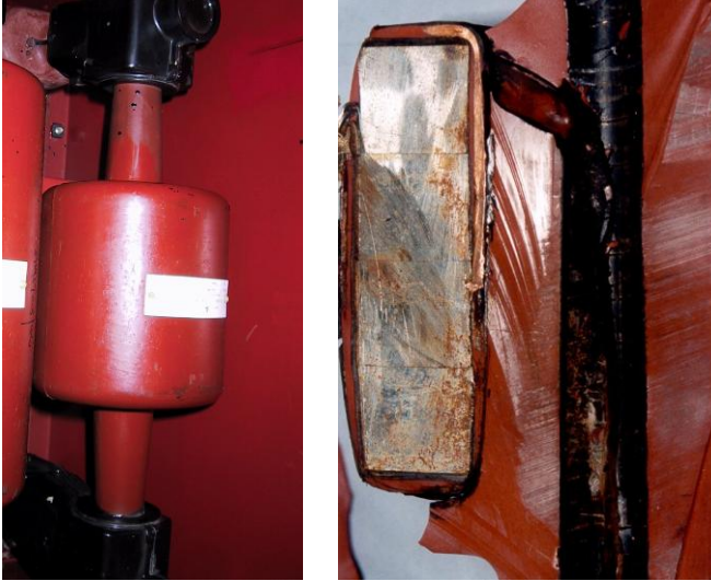
Figure 3 – Internal partial discharge
