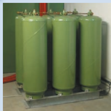
Oil Feeding Tanks for Low Pressure Oil Filled Cables
