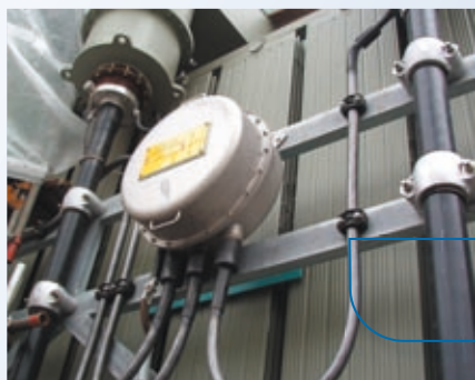
Link Box for Single Point Earthing Installed at Transformer Terminations
