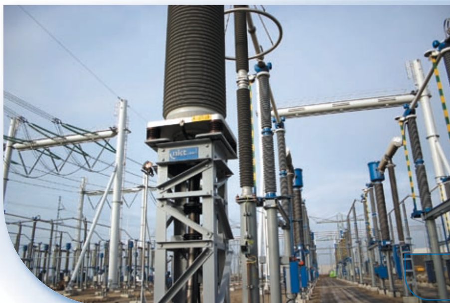
Outdoor Termination with Composite Insulator FEV 420-V
