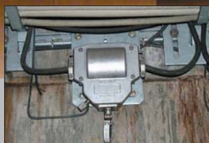
Express box for direct wiring
