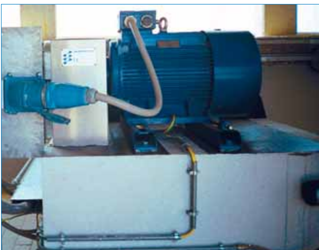
Typical connection of a cochlea motor.
