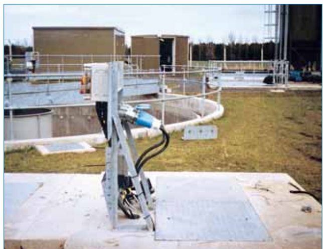
Typical connection of a submersible pump.
