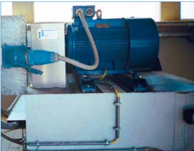
Typical connection of a cochlea motor.
