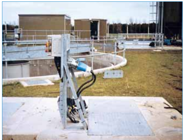
Typical connection of a submersible pump.
