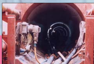
Mining and quarries
