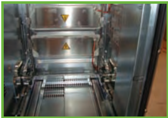
Figure 3: Retrofitted unit with new cell and breaker
