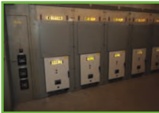
Figure 4: Front view of updated gear after replacement breaker project
