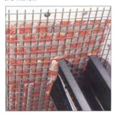
Place *KBS Sealbags* lengthwise and flat onto the wire mesh, layer after layer. The filling of tight spaces is accomplished as described above.
