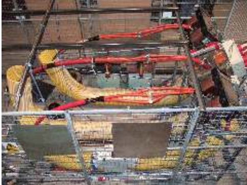
Picture shows Xlpe and Pilc 12kV Joints and Terminations undergoing type testing to BS 7888 and Cenelec standard HD 628 S1 and HD 629.1 S1
