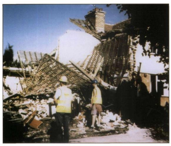
Figure I Aftermath of a gas explosion, following damage to an underground gas service pipe
