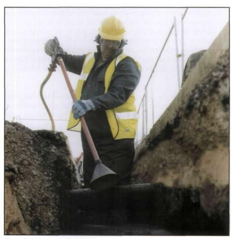
Figure 5 Using an air digging tool
