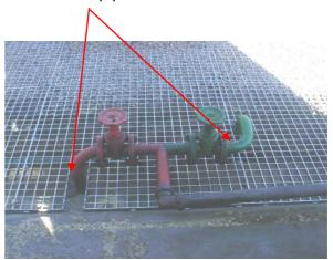
Cut half sections of grating where necessary
