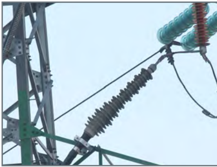
▲ Dry type outdoor termination angle mounted on a tower.
