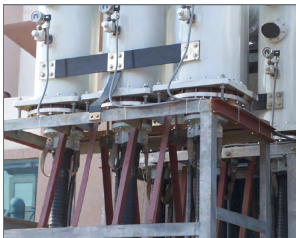
▲ PATR140-SF terminations installed in a GIS.
