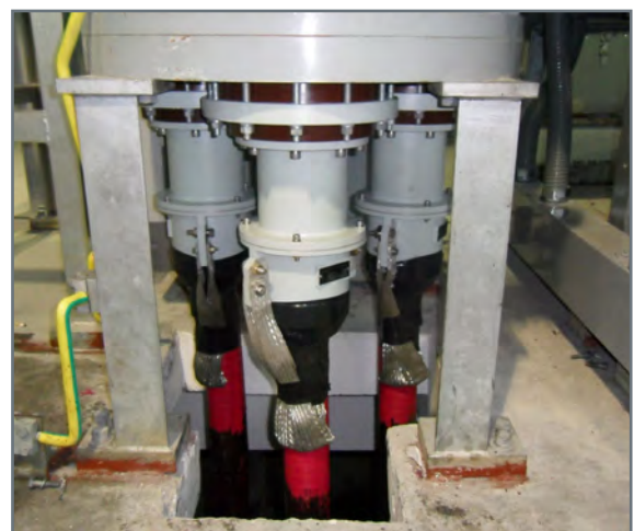
▲ SSC140-SF terminations installed in a GIS.
