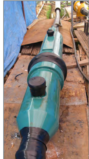
▲ Installation of premolded joint.
