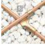
For applications where exothermic welding is not appropriate for creating permanent connections, compression connectors may be used.
