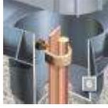
Where permanent connections are not appropriate, mechanical clamps offer the ideal solution. These are typically used on smaller scale installations where periodic disconnection for testing is required.
