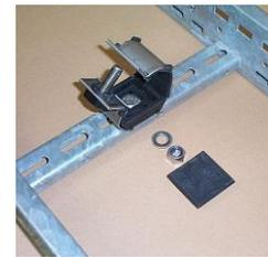
3) Replace the appropriate pad and install the cables.
