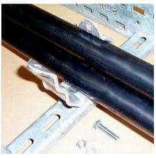
3) Replace the setscrew, sprung washer and nut and tighten.
