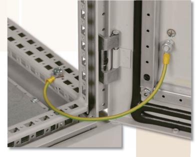
The frames of the Multi-Flex® series, MCS, MCD, MKS, MKD are equipped with contact washers so the earthing points can be mounted on any space available. To ensure that these earthing points will give you the desired protection, Eldon has verified their products by testing at the independent institute TNO in The Netherlands.
