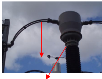
Figure 7.2A – Example of proximity of lower level equipment - Safety Distance to be maintained when applying portable Earthing Device(s) will be from the bottom of the CT housing not the conductor as indicated by the red arrows.
