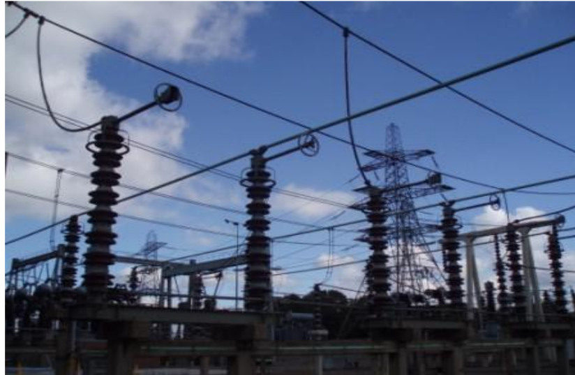
Figure 8.1A – End Rotating Post Busbar Isolators Arranged in Tandem
