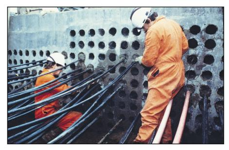
commonly run in ducts. Gas can accumulate in these ducts and seep[ into exchanges, sub stations, switchrooms etc. Therefore it is necessary to make an effective seal in the space between the cable and the duct. Spareways without cables also have to be sealed. Ducts below ground can also fill with water and this too would enter the exchange or sub-station. The seal has to prevent this. Water may exert considerable pressure and in a basement a two metre head is quite possible.
