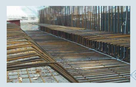
Earth Conductor in Concrete Foundation
