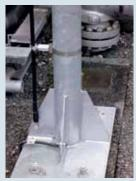
Connection of the HVI® conductor at the earthing terminal
