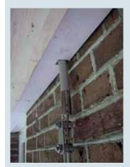
Fig. 3: Connection to down conductor system – Lead-through moulded board
