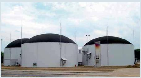
Biogas plant in Kerpen/Germany Protection of the fermenters – Air-termination masts with HVI® conductors
