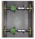
Figure 1: Wall bushing with formwork installation
