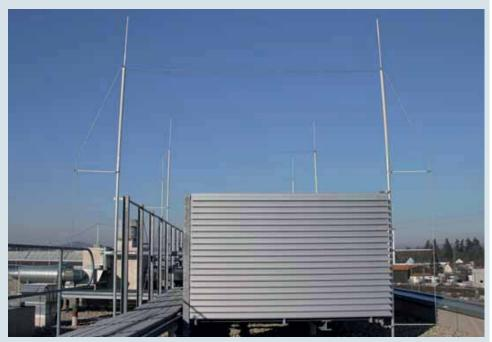
Isolated air-termination system for roof superstructures
