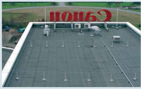
Supported air-termination system with spacers and concrete bases
