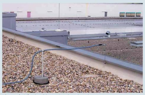
Adjustment of a HVI® conductor light connection to the metal-capped parapet
