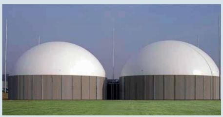
Protection of the fermenters with telescopic steel lightning protection masts
