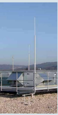
Isolated air-termination system for recooling plant with HVI® conductor in the supporting tube
