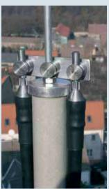
HVI® conductor – parallel leading with terminal clamp Part No. 301 329
