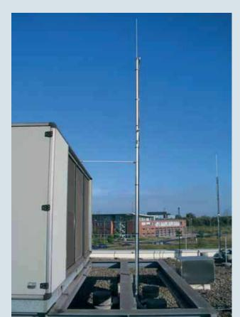
Isolated air-termination system at a roof superstructure with HVI® conductor
