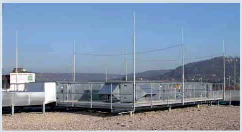
Isolated air-termination system DEHNiso-Combi and HVI® conductor in the supporting tube
