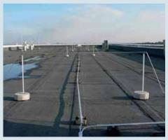
Supported air-termination system with spacers and concrete bases in the area of the electrical installation on the roof
