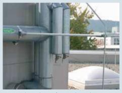
Spacer with attachment, fixing socket and tensioning strap
