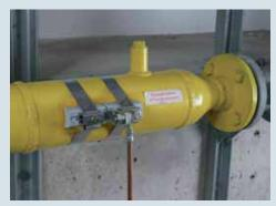
Figure 1: Pipe clamp for electrical contacting of pipes in explosion-hazard areas for implementing of lightning equipotential bonding according to EN 62305-3 (DIN VDE 0185-305-3)
