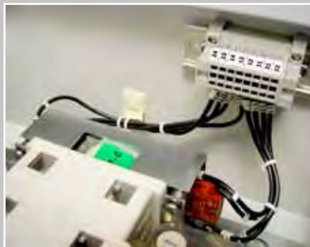
Interior view showing flag indicator and the auxiliary blocks wired down to terminals.
