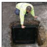
Lower chamber base into void and position as required.
