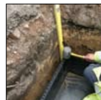
Ensure chamber is square and wall section is flush on base section.
