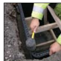
Ensure sections are fully interlocked.
