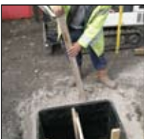
Make sure the chamber surround is well compacted.
