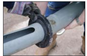
5 Remove gasket and cover plate from pole.
