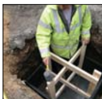
Place bracing inside of chamber.
