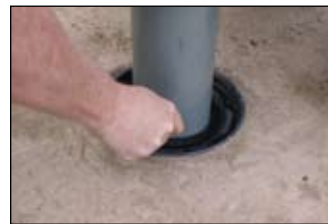
3 If necessary break seal between EPDM gasket and traffic signal pole.
