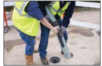
4 Lift pole out of socket.
