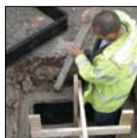
Ensure backfill is well compacted or concrete is tamped.
