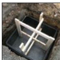
Place concrete or backfill around outside of chamber.
