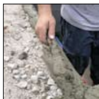
Place concrete surround around top of chamber.
