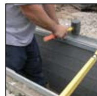
Adjust frame to level required.
