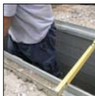
Site frame on to chamber/concrete surround.
