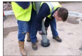
2 Raise cover plate to expose EPDM gasket.
