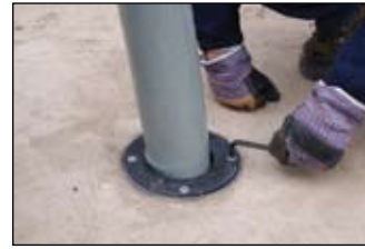
1 Remove cover plate locking bolts.
