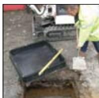
Ensure bottom of pit is level to allow base to sit correctly. Base should be compacted 10mm clean stone or lean mix concrete.
