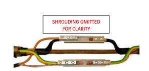
Apply an insulation wrap over the phase connector and secure using cable ties.
