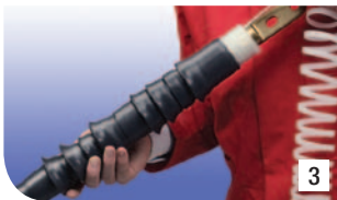
Begin to remove the inner core, allowing the termination to shrink down onto the cable
