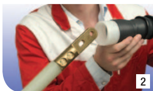
Place the 3M™ Cold Shrink termination body over the cable end and position at the correct point on the cable
