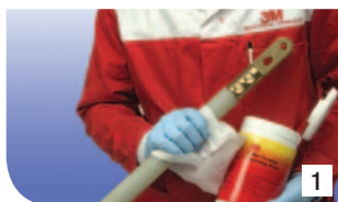
Prepare the cable as normal and clean with 3M™ Cable Wipes
