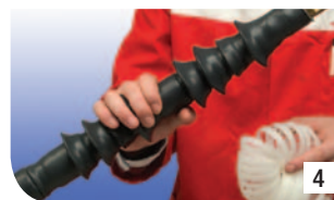
Once the inner core has been fully removed, the termination installation is complete!
