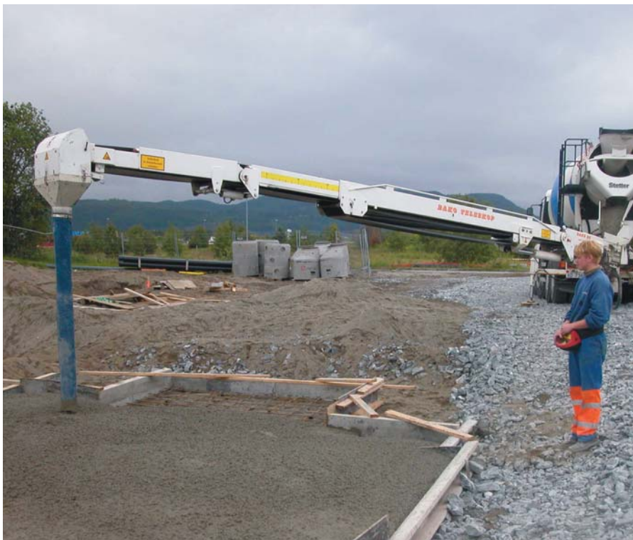
An MC-3-5 radio remote control being used to operate a cement mixing truck fitted with a conveyor belt.
