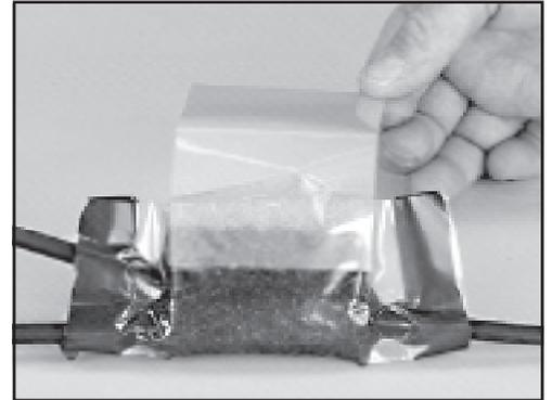
**3.11** Starting at top of looped film strip and proceeding downward, seal the loop together until top of mold is closed and the resin fills the mold completely.
