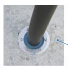
Single pipe transits: Dimension adaptable round seals for plastic pipes as well as steel pipes.
