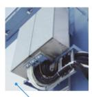
**I/C cabinets:** Neat and area efficient cable entry seals for top or bottom of cabinet.
